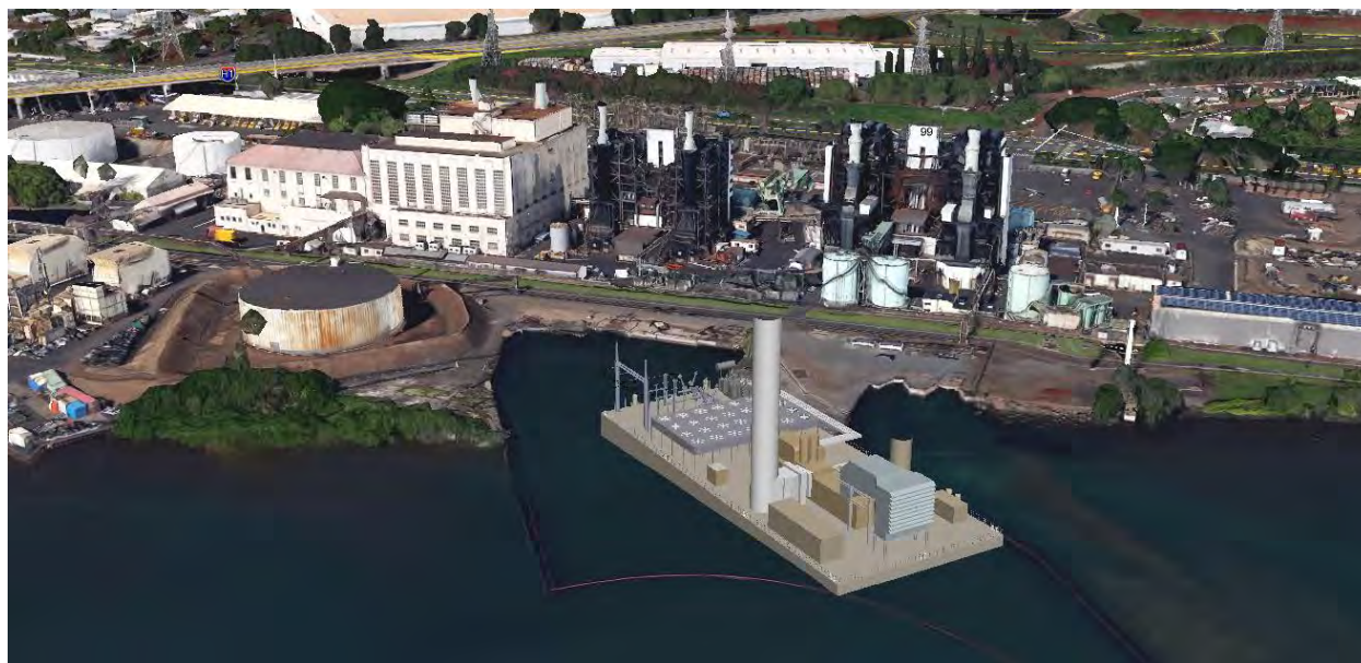
Figure D-45. Artist Rendering of Possible Power Barge at the Waiiau Generation Station
