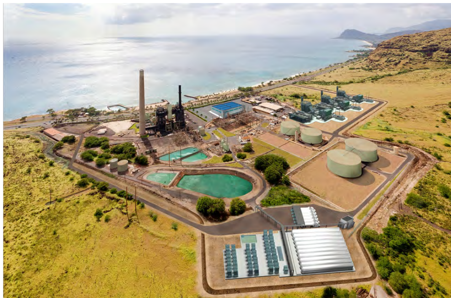
Figure D-4. Possible Kahe 3x1 CC with Removal of Kahe 1-4 (Artist Rendering)
