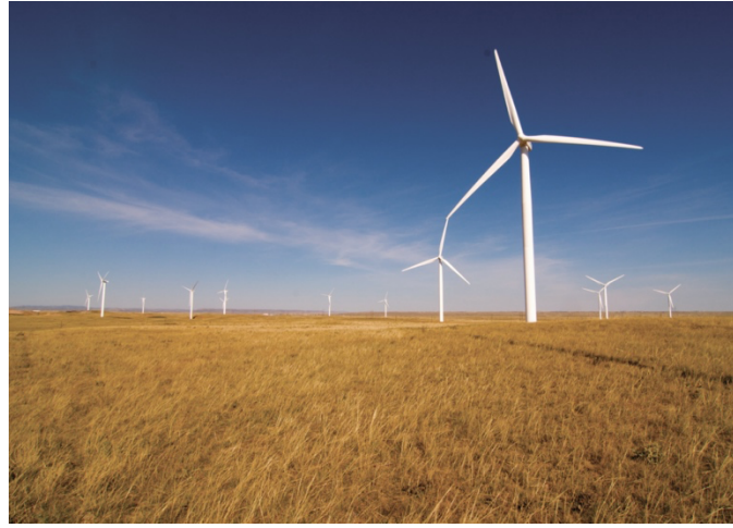
Figure 05-10. Happy Jack Wind Facility
