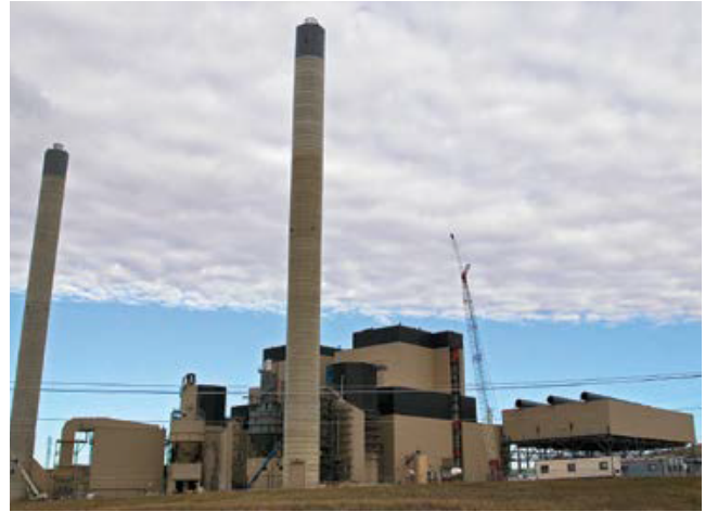
Figure 05-6. Wygen II and Wygen III Generation Facility
