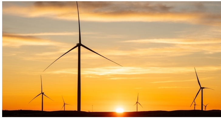
Figure 05-9. Corriedale Wind Facility
